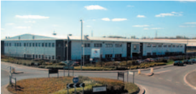
The AESSEAL® Global Technology Center is the largest of 47 facilities worldwide.
