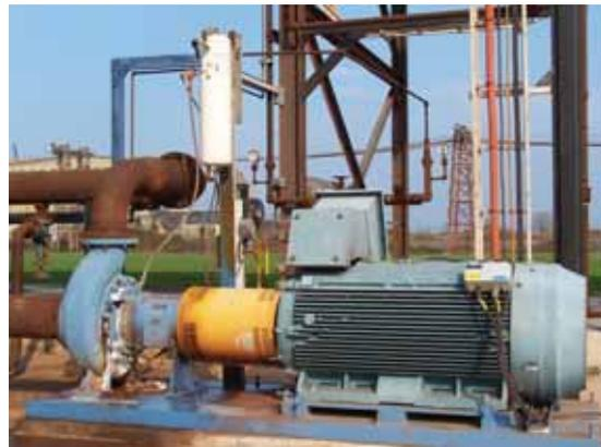
SSE25™ system with air-blast coolers installed in an alumina plant in Ireland.
